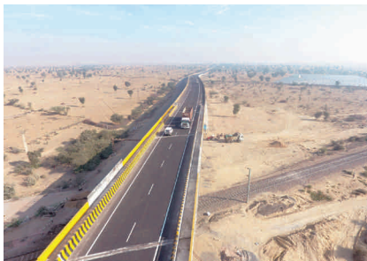
Railway over bridge in Bikaner-Suratgarh Section of NH-62 (earlier NH-15) in the state of Rajasthan for Ministry of Road Transport and Highways through PWD, Rajasthan
