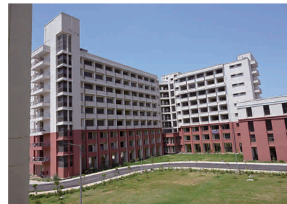
Construction of various buildings i/c residences of National Law University in Rajiv Gandhi Education City at Rai in Sonapat Distt, Haryana for PWD (B&R), Haryana
