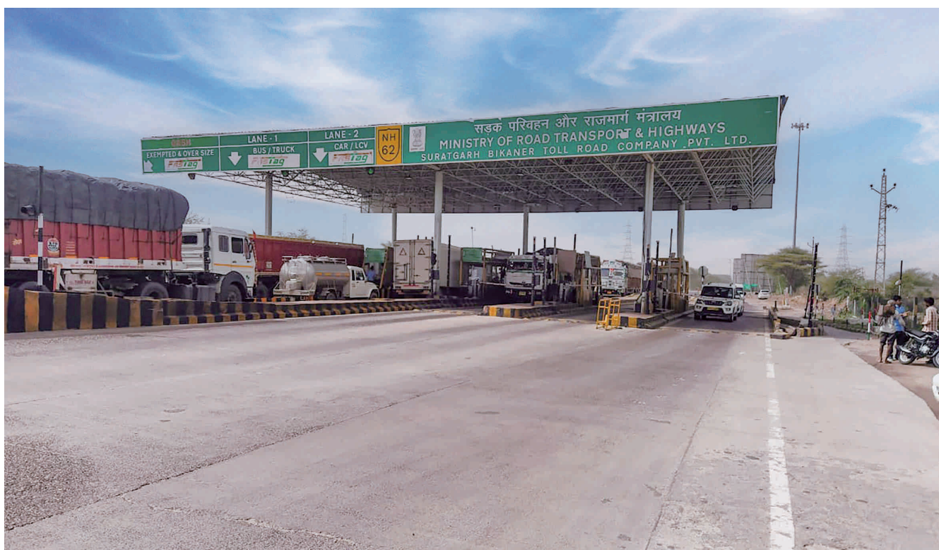
Development and operation of Bikaner-Suratgarh Section of NH-62 (earlier NH-15) in the state of Rajasthan for Ministry of Road Transport and Highways through PWD, Rajasthan
